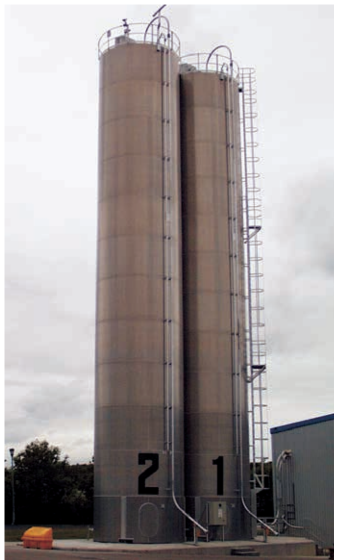
Figure 18 Storage silo for synthetic silica
